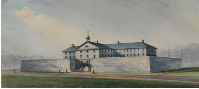
Figure 9: The Old Arch Street Prison 5
